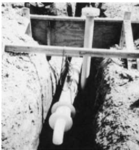
FIGURE B13.96 Example of a low-point leak-detection sump in a plastic gravity drain system.
