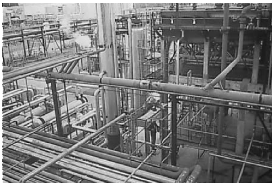
FIGURE C7.3 Typical process plant piping.
